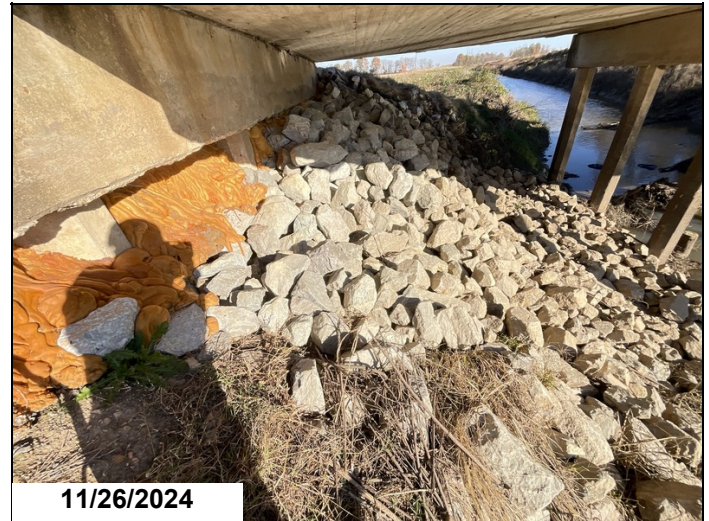
Bent 1 slope protection and expandable foam repair observed 11-26-2024
