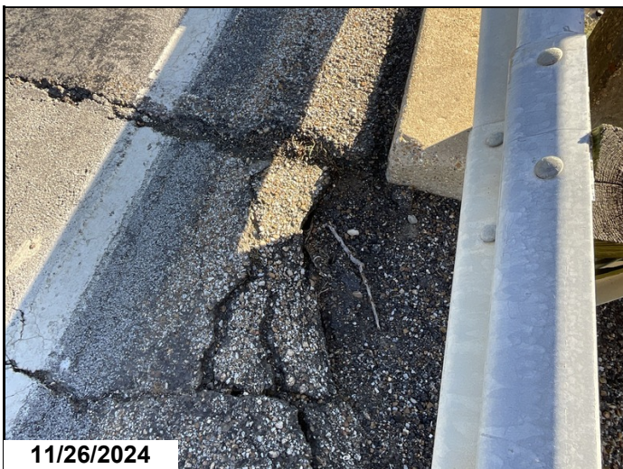
Bent 1 right approach roadway embankment repair observed 11-26-2024
